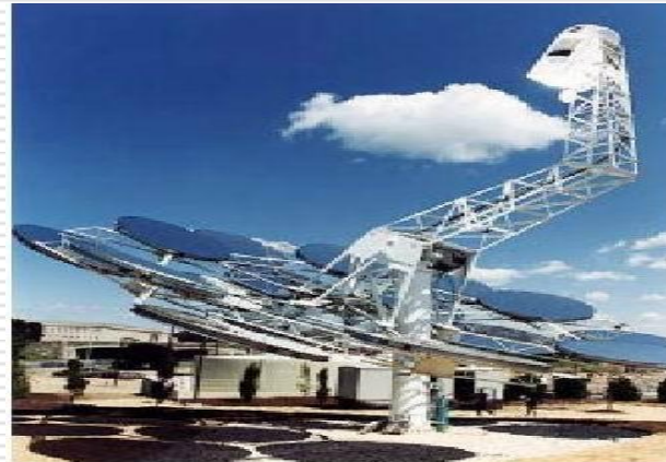
Figure 1. Dedication of the dish/Stirling system at the Pentagon in Washington, D.C. Shown in the picture are the concentrator and the STM 4-120 Stirling engine/generator package.
